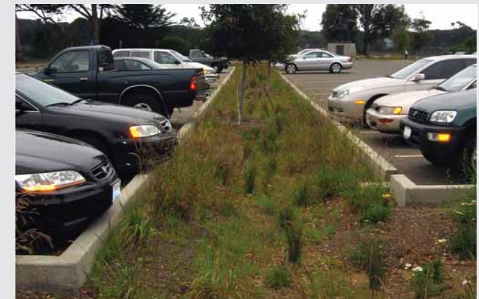
▼ The parking lot swale at Sunset Circle on Lake Merced accepts and treats runoff from the parking lot.
