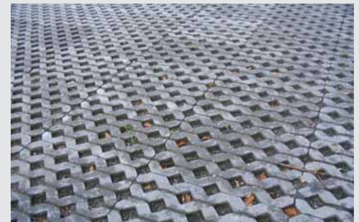
Some permeable systems allow stormwater to flow between pavers, as shown above. Others provide a solid surface without gaps, nearly indiscernable from traditional materials.
