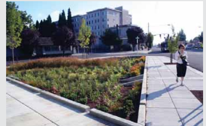
▲ Rain gardens are highly customizable, and can be designed to fit into any number of spaces within the streetscape. The above raingarden includes a channel, behind the pedestrian, to convey roadway runoff to the landscaped treatment area. (Source: Kevin Perry)
