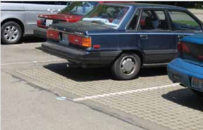
Existing paving materials can be replaced with permeable systems in retrofit situations. (Source: EPA Office of Water)
