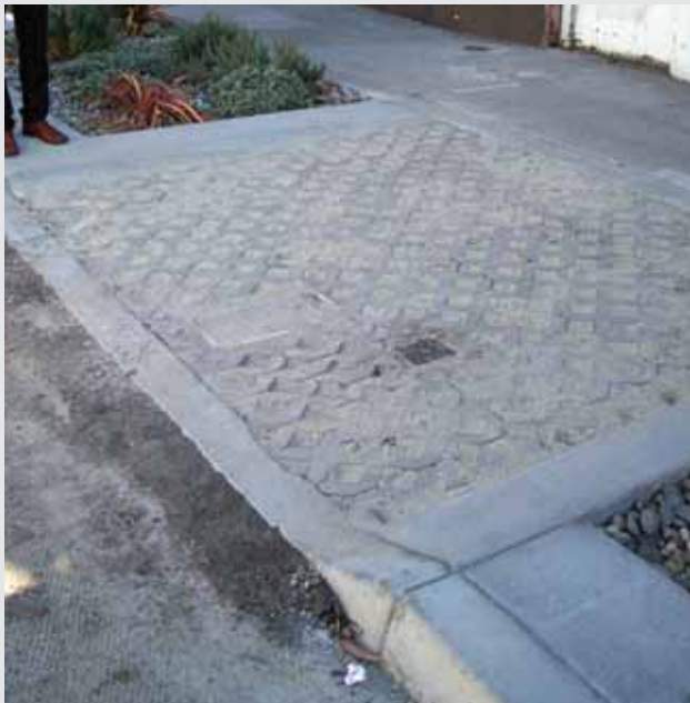
Bottom: Permeable pavers and other materials can allow stormwater to infiltrate through driveways and add a more attractive diversity of materials and textures to the streetscape.
