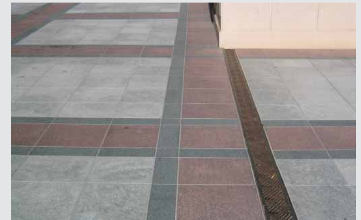
Channel covers can use attractive grates and can be integrated with other site design elements.
