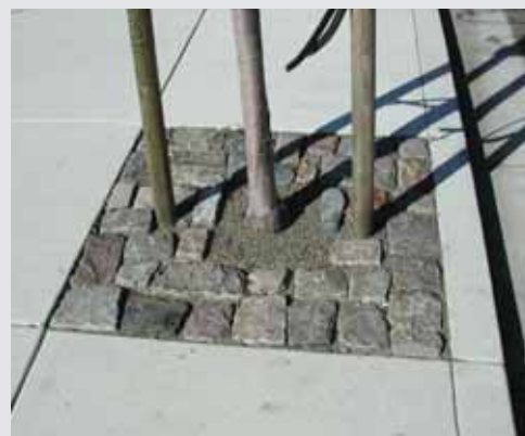
Using cobbles or other paving stones protects the basin and still allows root access to water
