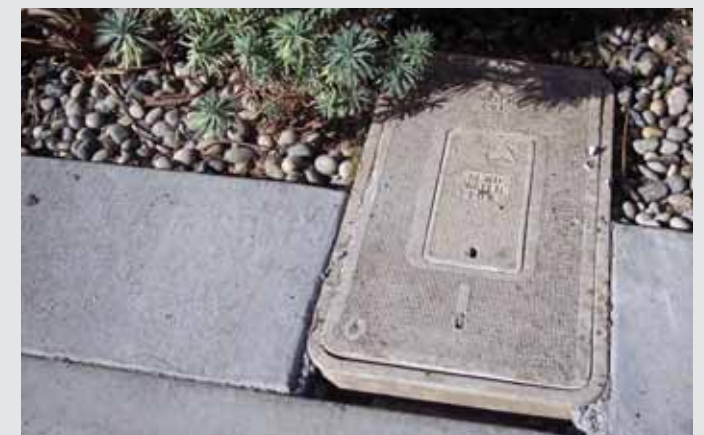
Utility vaults can be located within planting areas as long as they can be accessed.
