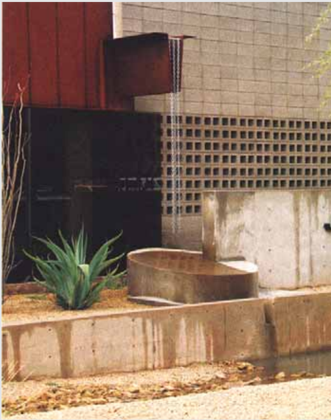
This attractive architectural planter and fountain is a disconnected downspout that drains to a planter with an infiltration trench below.
